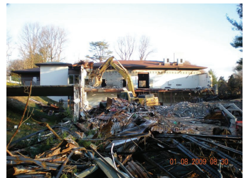
Figure 4 - Demolition of Existing Building
