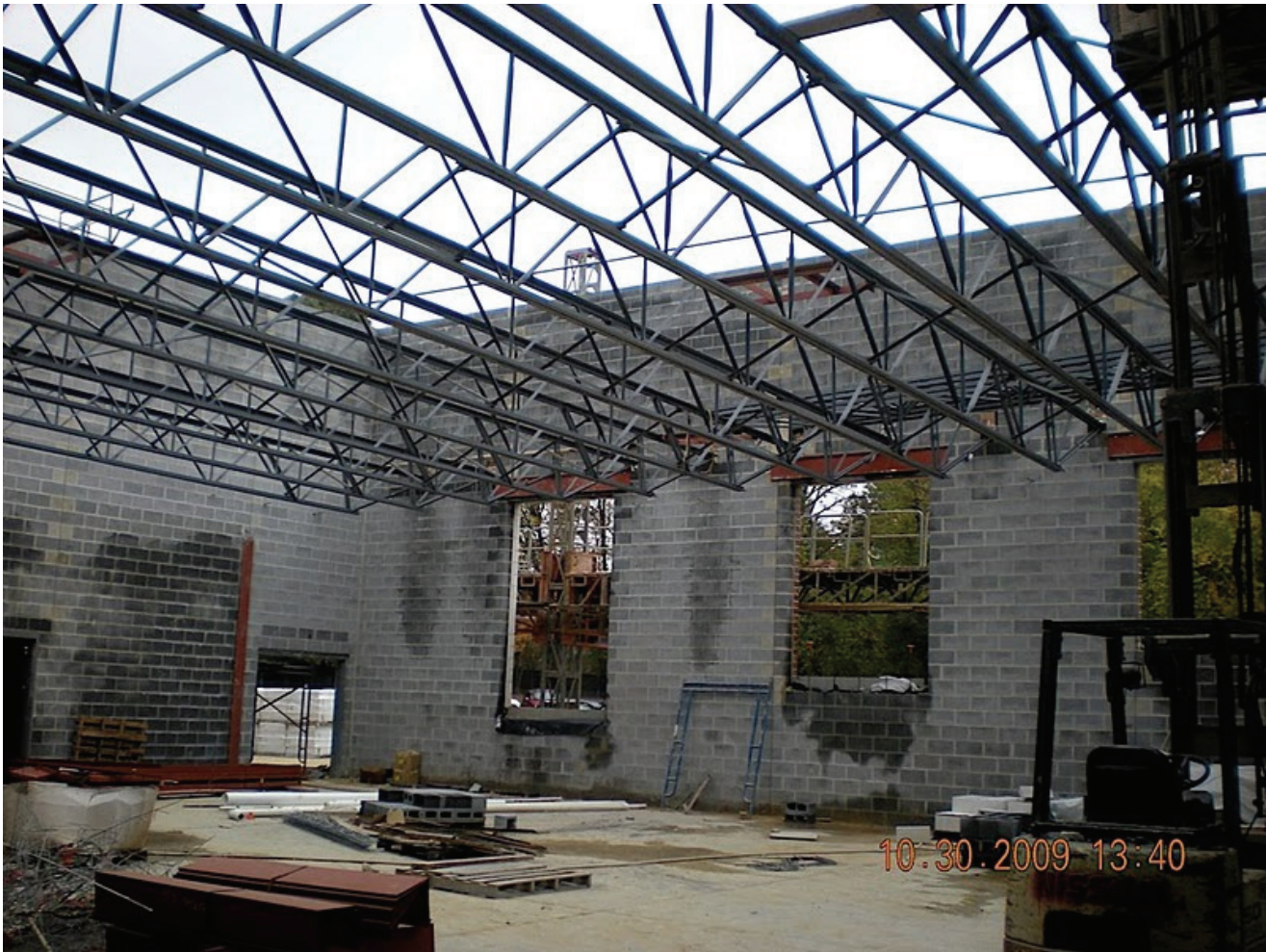
Figure 20 - Picture of Multipurpose Room
