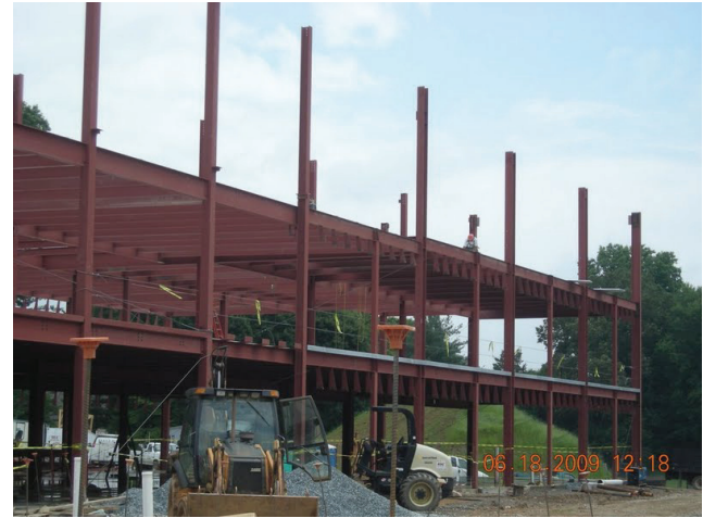
Figure 5 - Steel Frame at Carderock
