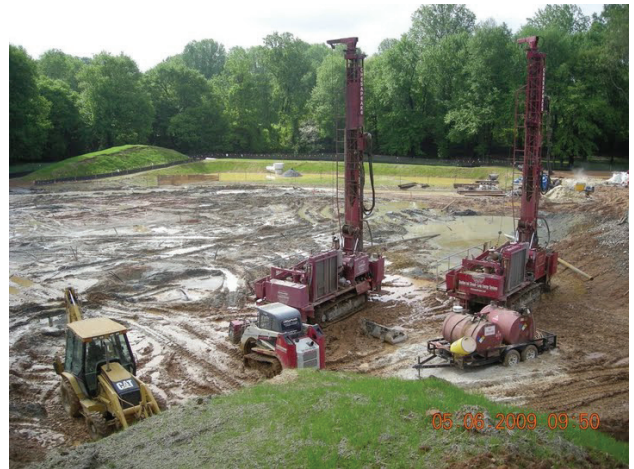
Figure 7 - Geothermal Well Drilling
